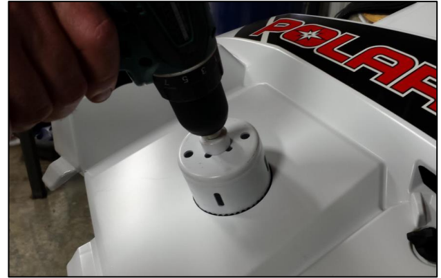
10. Drill a pilot hole in the center of the X, then using a 3" hole saw, drill a hole.
