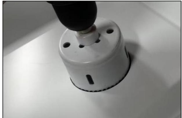
4. Using a silver marker or pen, mark the center of the fan opening. Remove faceplate and rivets. Using a 3" hole saw, cut out the fan opening using the center lines as a guide. De-bur the holes you have drilled.
